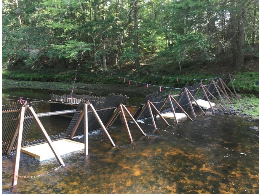
Figure 2. Upstream view of the operational picket weir. Collection box is central and floating panels are visible in the foreground.
